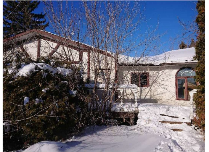
One of the buildings to be demolished
