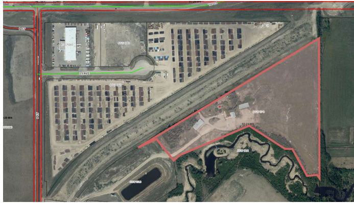
Lukas property, aerial view
